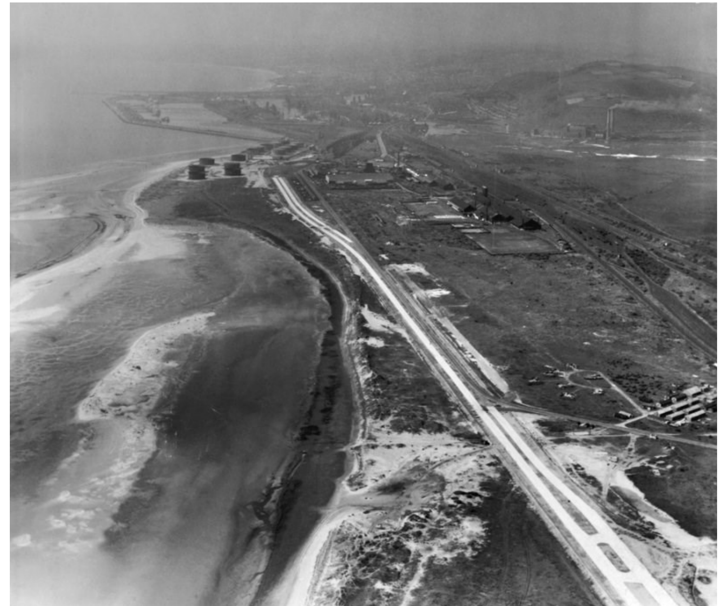
Fabian Way, or Jersey Marine Road, now A483, was constructed between May 1946 and September 1950. Amazon now lies to the right of the dual carriageway and the bay area was reclaimed for petro-chemical tanks, now the Swansea University Bay Campus.
